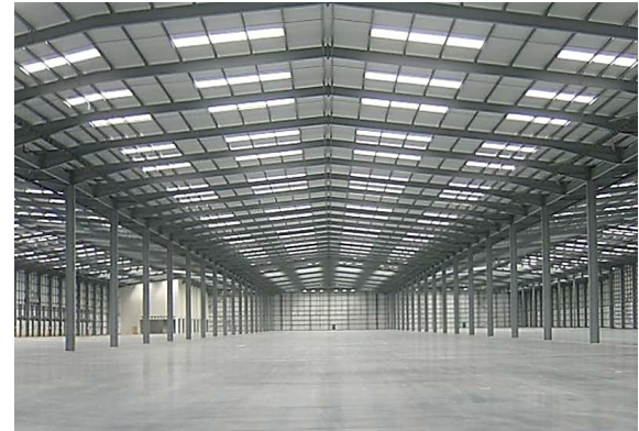
MULTIPURPOSE SHED STRUCTURE
